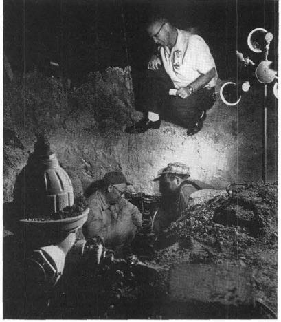
NEW VALVE to control fire hydrant near Bldg. 893 is installed at night by personnel of Section 4514-3. Caulking the valve are Conroe Wyman, left, and Manuel Sanchez, while A. O. Butts, one of the supervisors of Section 4514-3, waits to inspect final seal.
